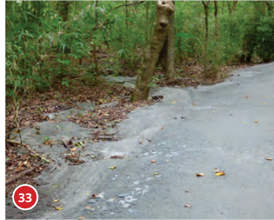
• Stormwater runoff eroding trail
