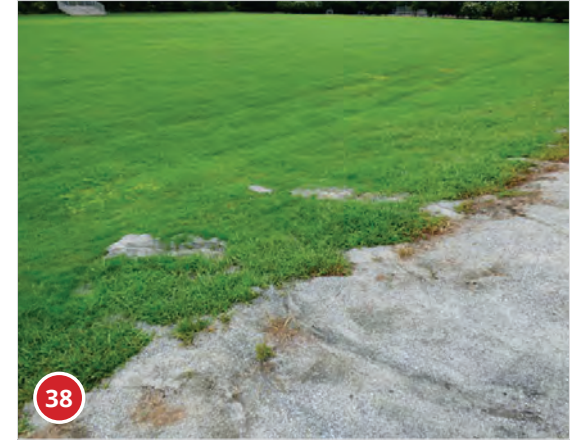
• Stormwater runoff eroding trail and moving sediment
